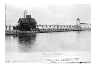
The postcard shows the old lighthouse (built in 1889) on the North pier, around the year 1900. The fog signal building was equipped with a 10" diameter steam whistle (mounted in the box on top of the building)
